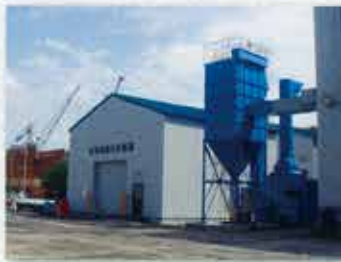
▲ 塗料保管庫棟 (114m)
